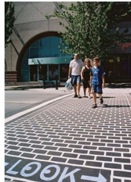
DuraTherm®, an inlaid thermoplastic crosswalk treatment.
