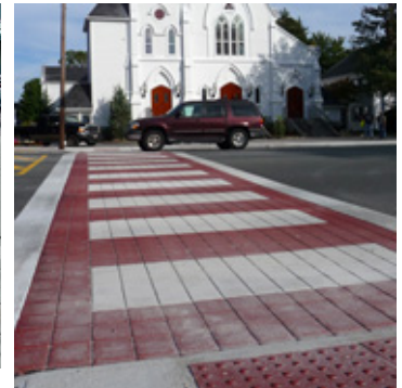
StreetPrintXD®, a heat-stamped, colored asphalt treatment.
