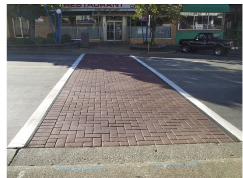
A traverse pattern is painted on the street to define the edge of this special crosswalk treatment.
