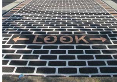
A “look” stencil may be incorporated into the crosswalk to encourage pedestrians to look both ways, particularly at unsignalized intersections.
