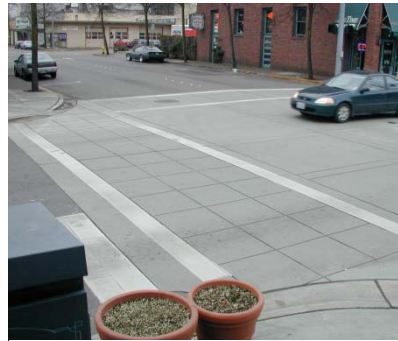
Stamped concrete with traverse pattern defining the crosswalk edge, and an advanced vehicle stop bar.
