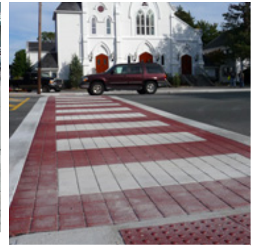
StreetPrintXD®, a heat-stamped, colored asphalt treatment.
