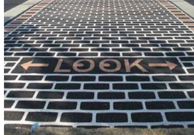
A “look” stencil may be incorporated into the crosswalk to encourage pedestrians to look both ways, particularly at unsignalized intersections.
