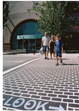
DuraTherm®, an inlaid thermoplastic crosswalk treatment.
