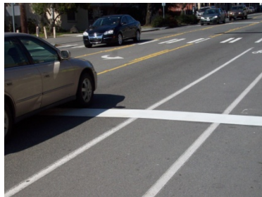
An advanced stop line may be installed at unsignalized crosswalks to provide for adequate stopping and sight distance.
