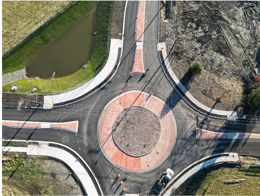
Figure 4- 244th Ave / Roosevelt Ave Roundabout Intersection Improvements
