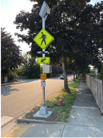
Figure 3-Warner Ave RRFB Crossing
